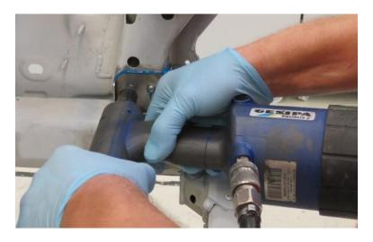
2. Fit the side rivets using the compressed air riveter.
